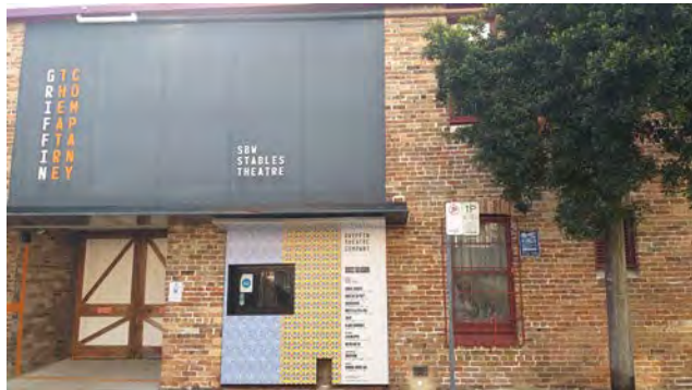
Figure 90: View of steel awning demarcating the main entrance and box office ticket window facing Nimrod Street.
