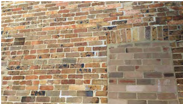
Figure 107: Brick infilled windows and different designs of metal ventilation grilles found on main facade facing Nimrod Street.
