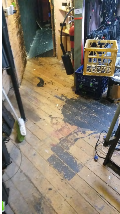
Figure 139: Bio Box room. Source: TZG Architects, 2022.
