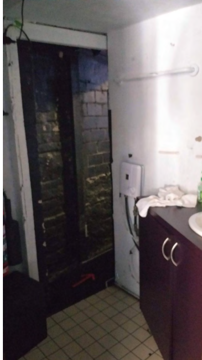
Figure 144: Backstage bathroom with corridor leading to the stage. Source: TZG Architects, 2022.
