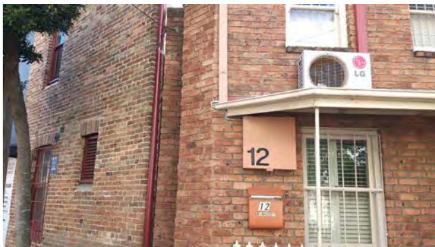
Figure 109: View of junction between the SBW Stables Theatre and neighbouring terrace house at 12 Nimrod Street. The two buildings are separated by a narrow brick wall.
