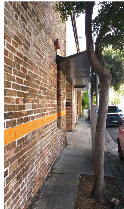
Figure 104: View along Nimrod Street of steel awning above the main entrance to the theatre.
