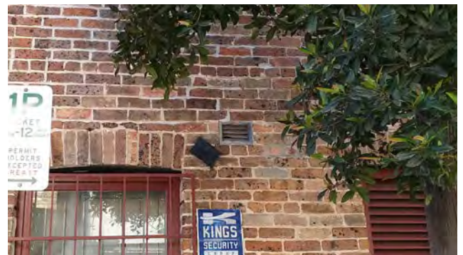
Figure 110: Metal element possibly associated with original stable doors (now removed) on main facade.
