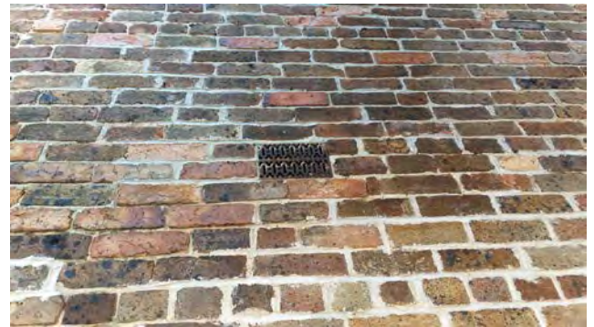
Figure 108: Metal ventilation grille and evidence of repointing on main facade facing Nimrod Street.
