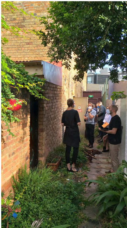
Figure 99: View of rear lane looking west towards Nimrod Street with brick boundary fence for terrace house seen abutting the external wall of the theatre.
