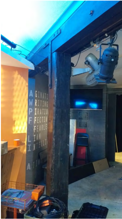
Figure 121: View of timber column and beam supporting the upper levels and separates the foyer and bar areas.
